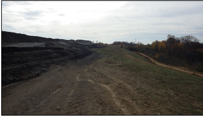
Photo 10 Stormwater ditch maintenance at toe of CCRs near Point 15, looking south. (Appendix A)
